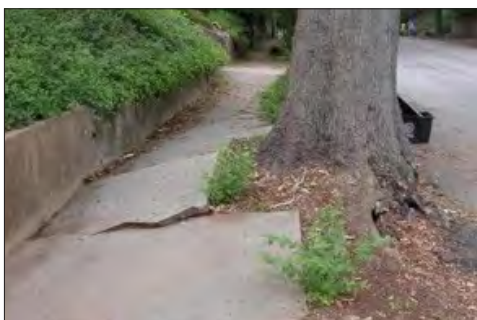
Damage to sidewalk
