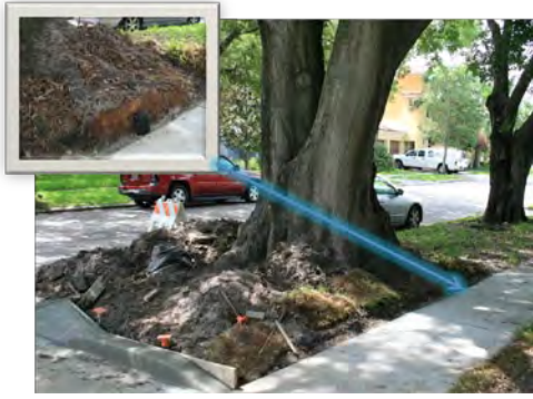
Sidewalk repair and damage to tree
